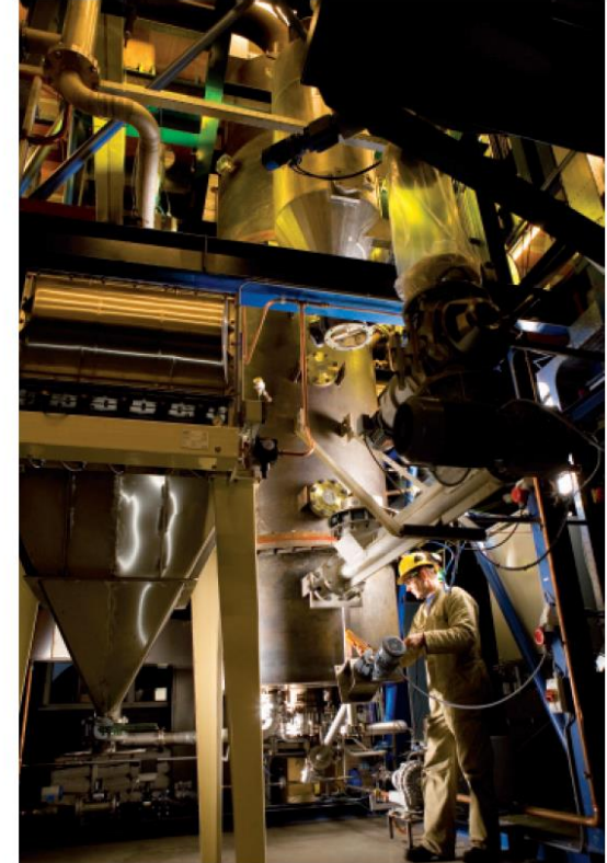
800 kW MILENA pilot gasifier
