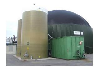
Digestion =>  $\sim$ 40% CO<sub>2</sub> +  $\sim$ 60% CH<sub>4</sub>
