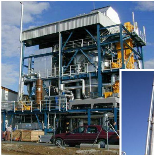
RME-scrubber, Güssing (A) CHP 2 MW e
