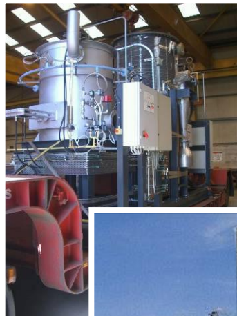
Biomass Engineering (UK) 250 kW e
