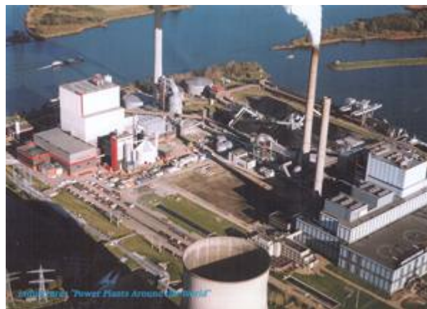
2x600 MW e coal boiler, Geertruidenberg (NL)
