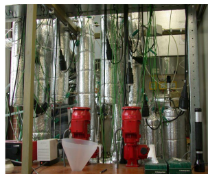
OLGA tar removal
